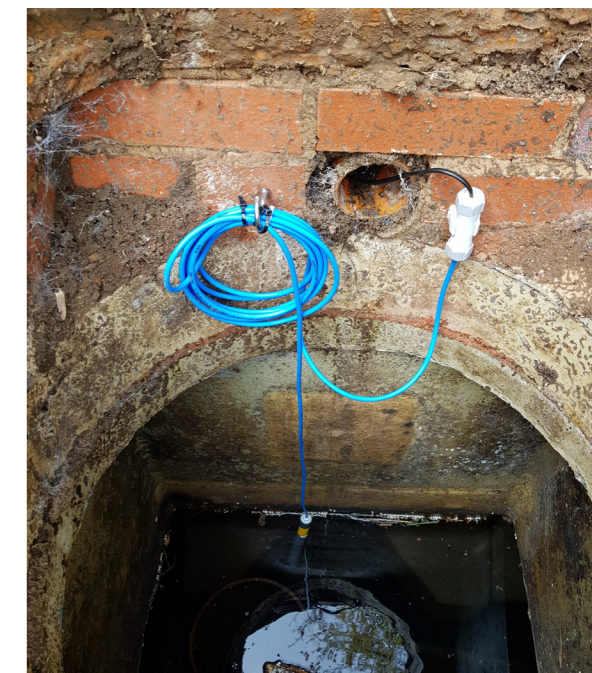
Top: the web-based Smart Sensor monitoring dashboard. Middle: a GSM modem which can be connected to mains or solar power. Below: a smart oil separator sensor being installed.
